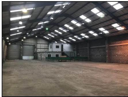
The above photograph is internal Unit 2.
